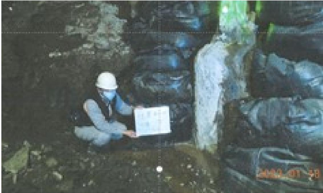
(b) Emergency stabilization of sliding with sandbags and water sealing with CCP (2)
