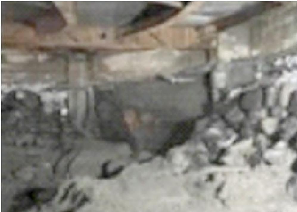
Figure 21. Sliding failure of rock debris from shear bands observed in the side walls of the Fongcai-520 high-rise building's basement.
