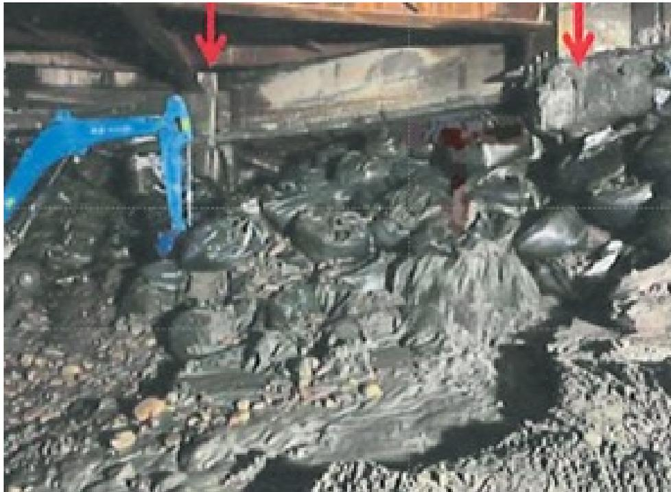
(a) Emergency stabilization of sliding with sandbags and water sealing with CCP (1).
